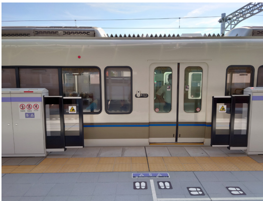
Platform Door Umekoji Kyotonishi Station
